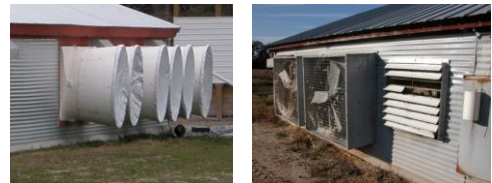
High Efficiency Cone Fans vs. Less Efficient (Box) Fans
