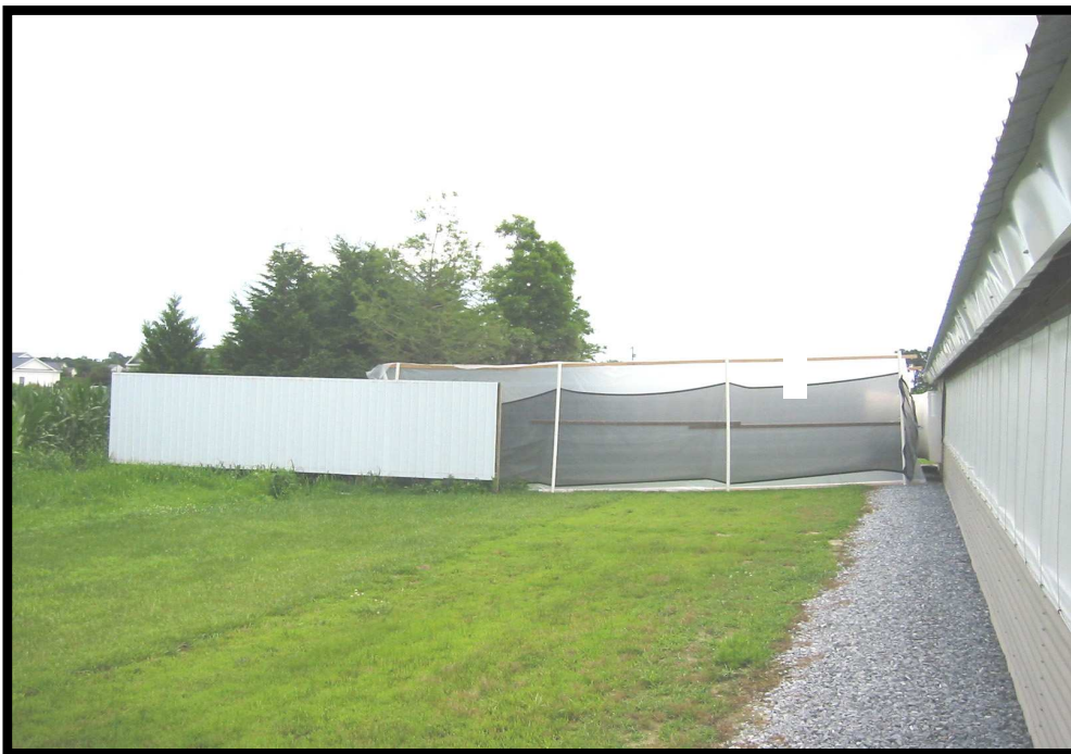
Figure 3. Wing-walls between fans and vegetative buffer installed to minimize influence of crosswinds on air quality measurements.
